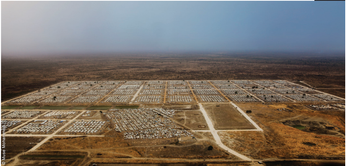
The expansion plan included land that was already spontaneously occupied by camp residents. Careful phasing of major upgrading works was required, as the whole site needed to be upgraded.
