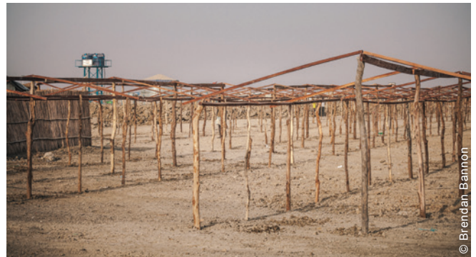
Shelter frames were built by contractors.
